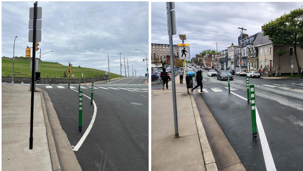
Figure 5. Curb extensions using low cost materials (Credit: Contributed (DF, and DB))
